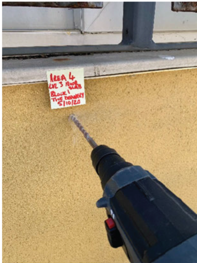
View of inspection location
