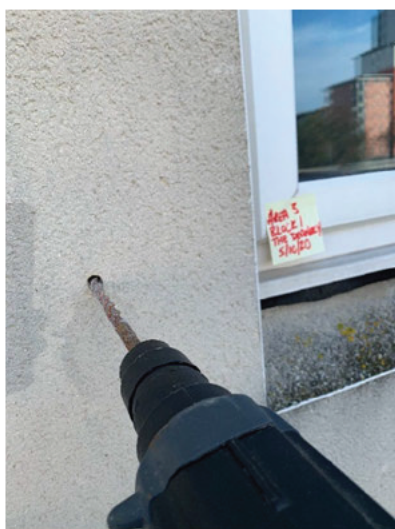
View of inspection location
