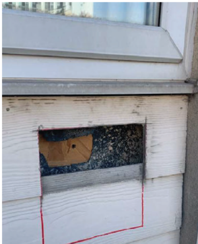
View of inspection location
