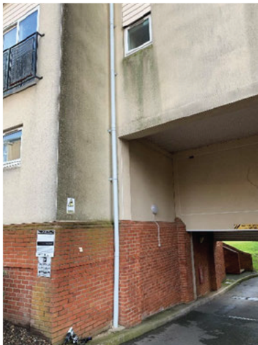
View of inspection location
