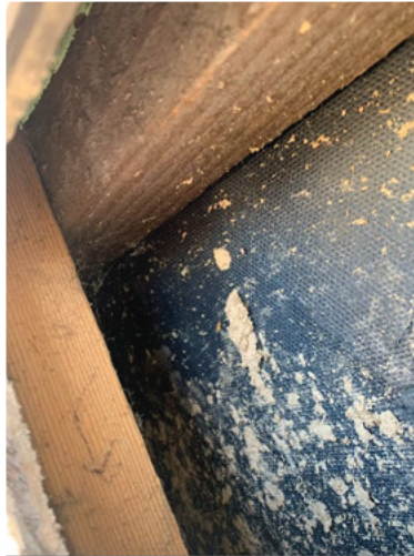
View of timber frame behind fibre board plank system
