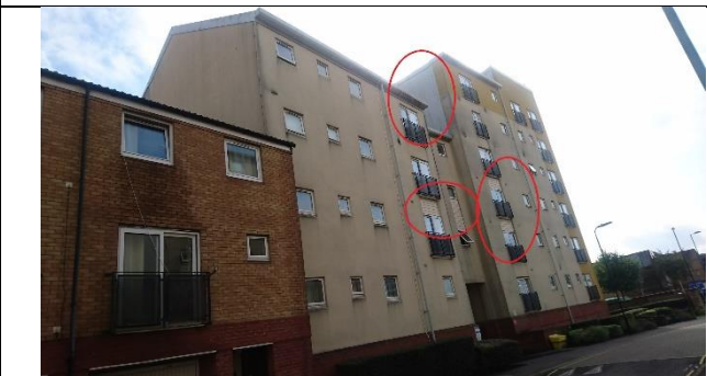
Suspect cladding
