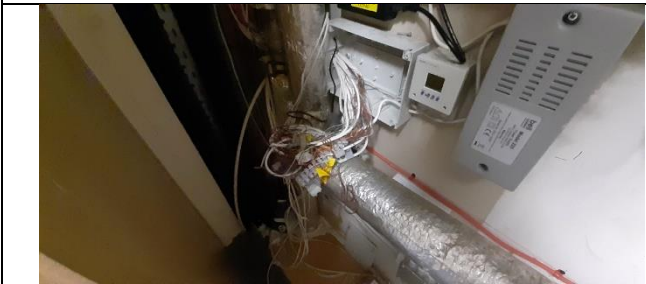
Evidence of poor cable management
