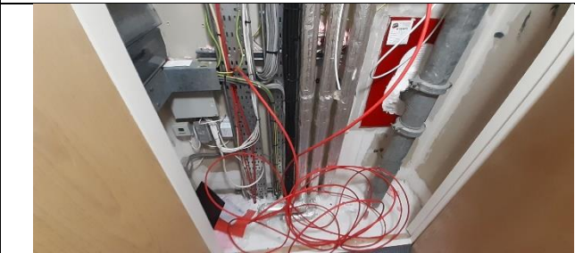
Evidence of poor cable management
